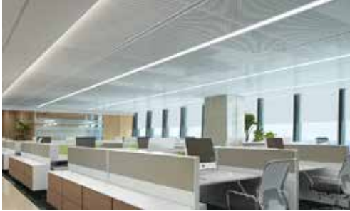
İç Mekan Aydınlatma Indoor Lighting
