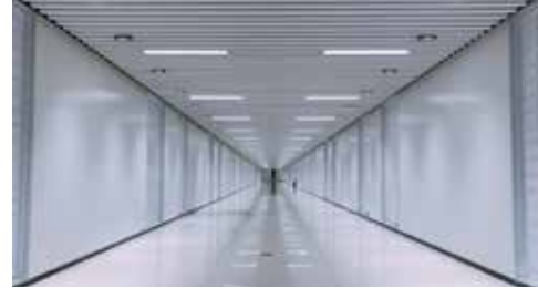
İç Mekan Aydınlatma Indoor Lighting
