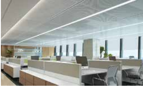
İç Mekan Aydınlatma Indoor Lighting
